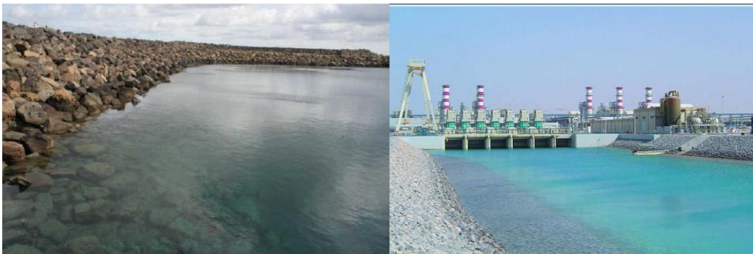
Figure 6: Examples of open intake basin protected by breakwaters [7]
