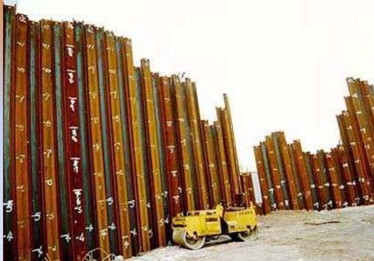
Sheet piles marked for driving
